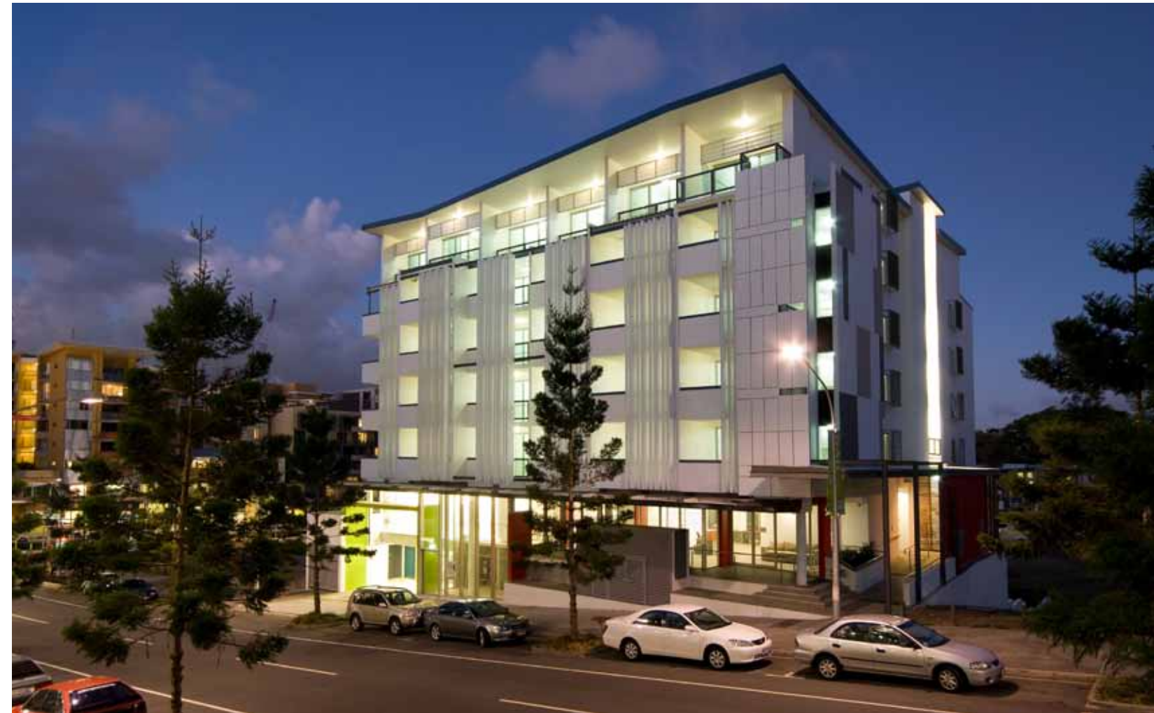
Tom Burns Place, Kelvin Grove Urban Village. A mixed use development comprising 2 commercial tenancies and 56 self contained apartments completed in 2007. Brisbane Housing Company proudly acknowledges the support received from the Queensland Government, Brisbane City Council and our Community Shareholders including Queensland Shelter.
